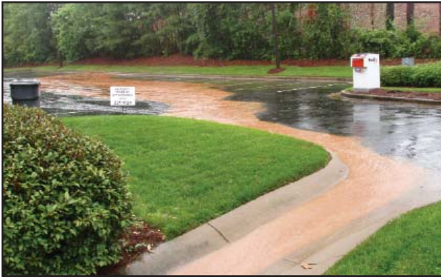
Figure 2.13 - Offsite impact from a neighboring construction site.
