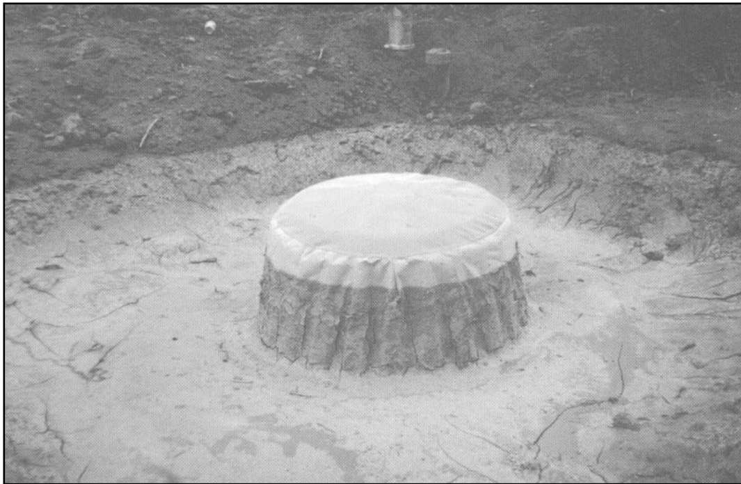
Figure 6-28.7 Alternative Inlet Sediment Trap
