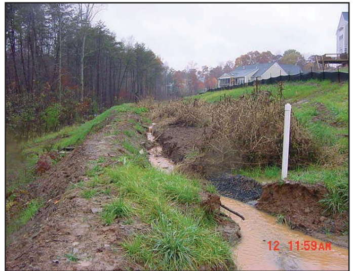
A major issue with conversions is timing. Premature installation of the post-construction practice can result in damage from construction sediments.
