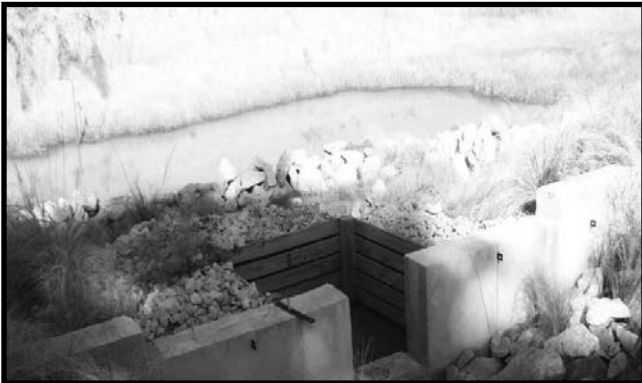
Example of Slotted Board Dam
